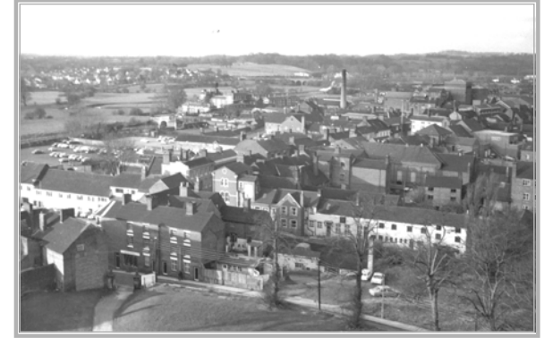
➤ 1975 Photo of Stone Town Centre taken from St. Michael Church.
