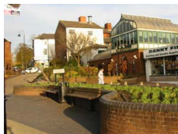
➤ Refurbishment of Earl St.Vincent Square.
