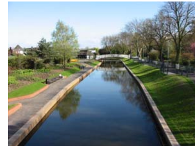
➤ P65: Quality paving along towpaths to create excellent riverside, Stafford Victoria Park.
