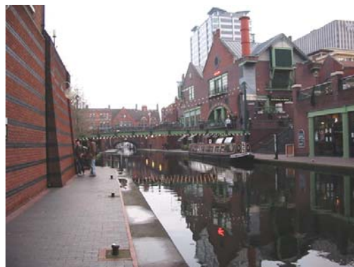
➤ A good mixed of uses (including retail units, restaurants and bars) along canal, Brindley Place.
