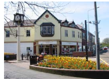
➤ P12: Corner detailing, Gaolgate retail development, Stafford town centre.
