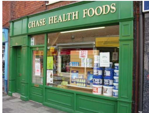
➤ P83 & 84: Shop-fronts should be well designed and fit into the Stone Conservation context, Stafford town centre.
