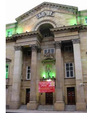
➤ P78, 79 & 80: Lit up historic building, Manchester City Centre.
