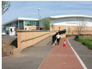
➤ P37: Introduce ramps at towpath to allow people with disabilities access to canal, Stafford.
