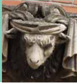
Oddfellows Hall, Greengate Street
