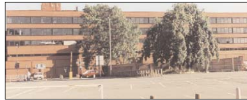
View across the site towards South Walls
