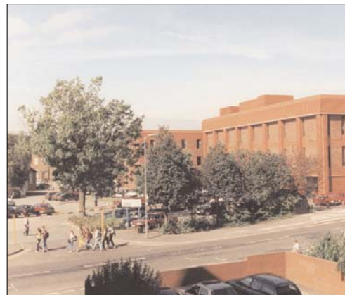
View of Magistrates Building
