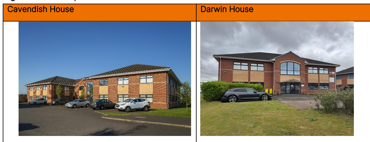
Figure 5.12 Examples of out of town offices
