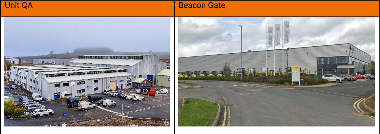
Figure 5.8 Examples of industrial/warehouse units Beacon Business Park
