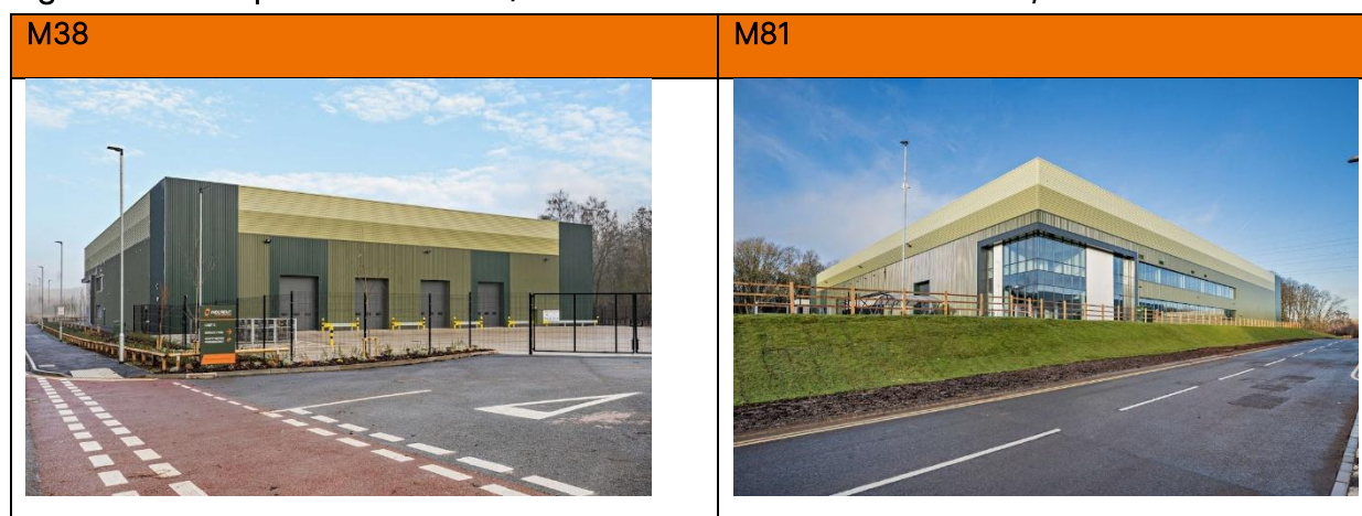
Figure 5.5 Examples of industrial / warehouse units at Indurent Park, Meaford
