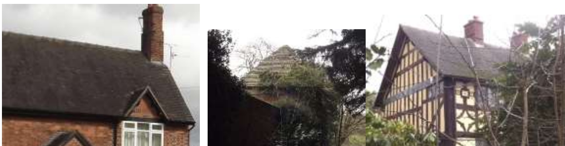
Figure 13 Fish scale design roof tiles to School House, pyramidal roof to the Garden House and decorative panels and projecting purlins to Olde House Farm
