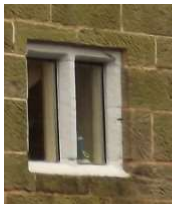
Stone mullion windows
