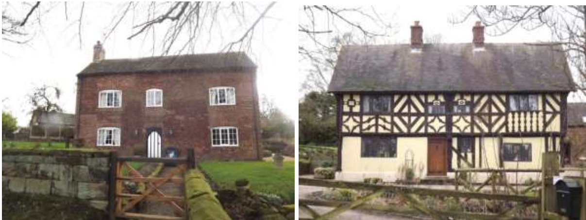
Figure 17 Rocklands and Olde House Farm
