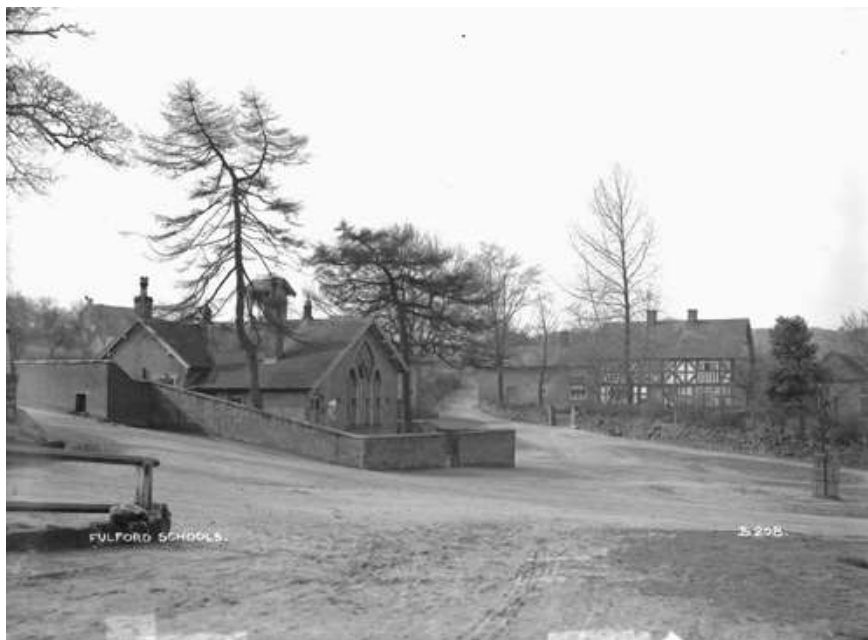
Figure 4 The National School with Olde House Farm in the background (staffspatrack)
