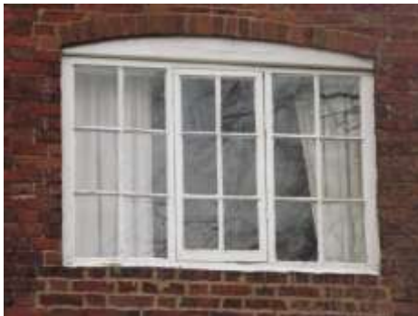
Side opening timber casement windows
