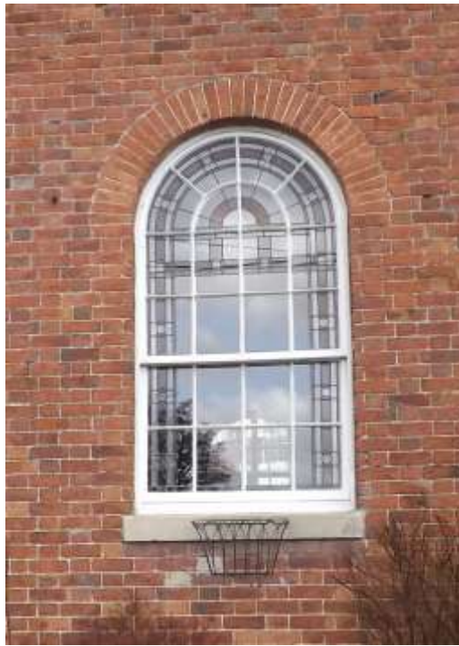
Arched vertical sliding sash windows to former Wesleyan Chapel
