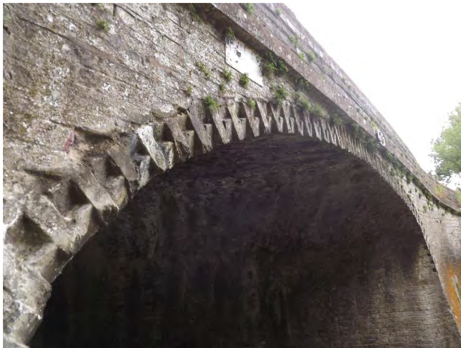
Figure 30 Brick detailing to Roving Bridge No.26
