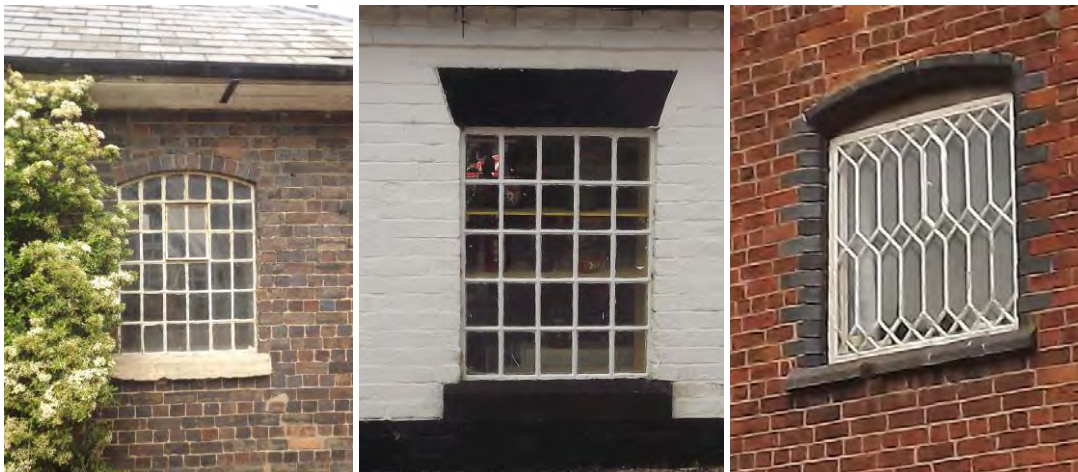
Figure 18 Multi-light, iron framed windows
