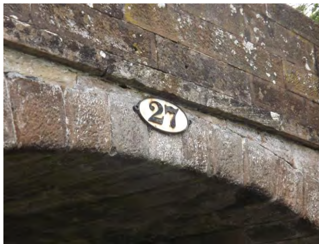
Figure 13 Cast iron bridge plates
