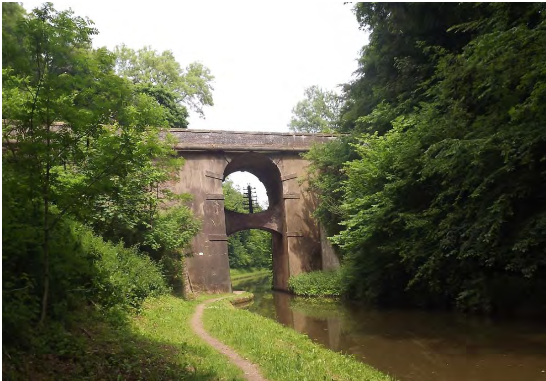
Figure 10 High Bridge (39) displays an unusual double arch
